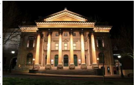
Capital Theatre 50 View St Bendigo – Former Masonic Building
