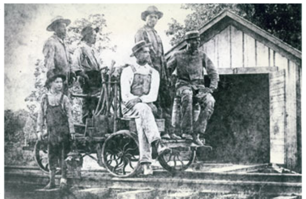
One of the original railroad crews from the 1900s
