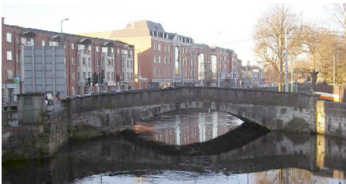
Recent View of Baal's Bridge, Limerick
